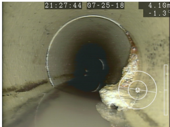
Figure 22: Calcite Buildup (4.1m from MH 42 towards MH 34)
