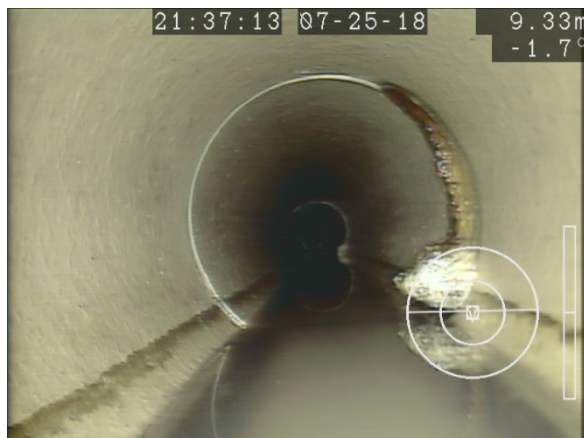
Figure 23: Calcite Buildup (9.33m from MH 42 towards MH 38)
