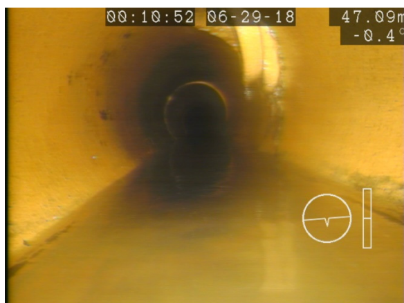
Figure 15: Calcite Buildup (47.1m from MH 5 towards MH 4)
