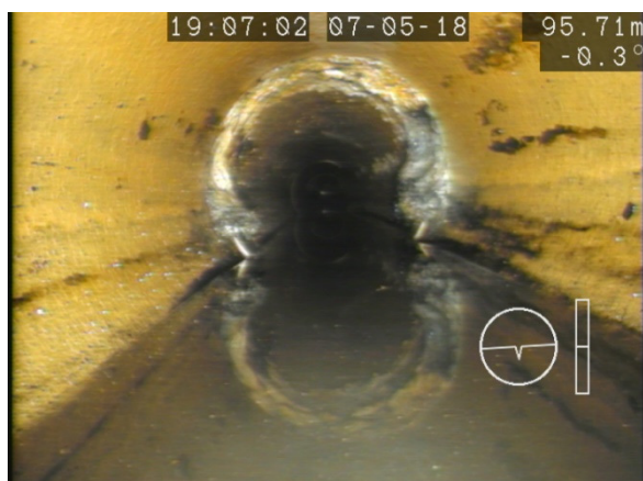
Figure 30: Calcite Buildup (95.71m from MH 18 to MH 29)
