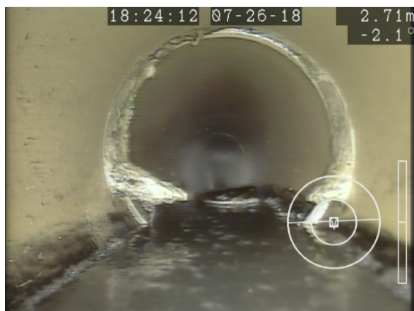
Figure 34: Calcium Buildup (2.7m from MH 35 towards MH 31)
