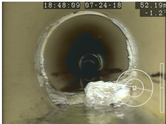
Figure 25: Calcite Buildup (55m from MH 28 towards MH 29)
