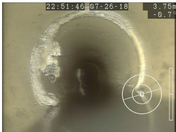
Figure 32: Calcite Buildup (3.75m from MH 22 towards MH 19)
