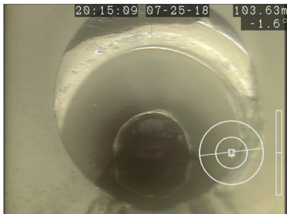
Figure 29: Offset in Pipe Just Outside Manhole (MH 35)
