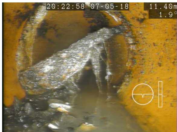
Figure 5: Large Debris Lodged in Pipe (11.4 m from MH 17 toward MH 18)
