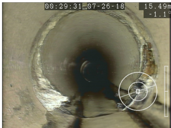
Figure 17: Calcite Buildup (15.5m from MH 32 towards MH 31)
