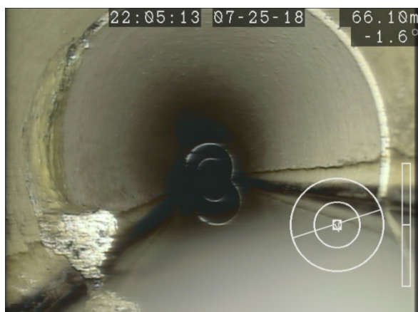
Figure 21: Calcite Buildup (66.1m from MH 38 towards MH 42)
