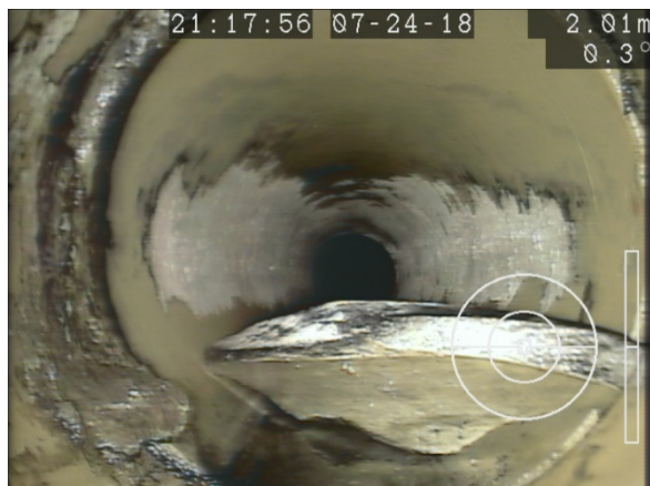
Figure 8: Broken Piece of Clay Pipe (MH 22)
