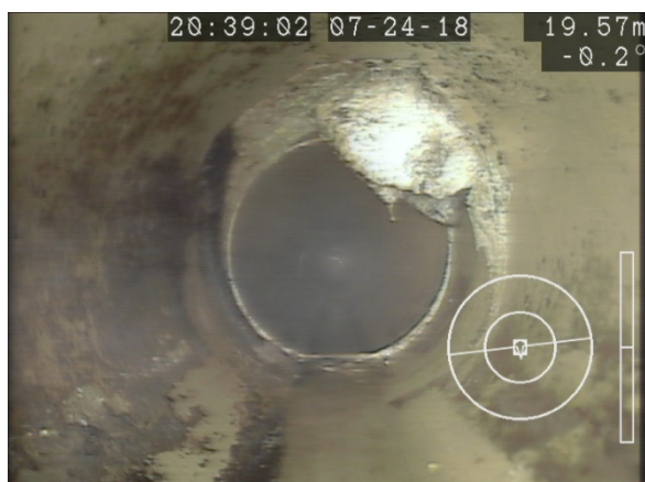
Figure 9: Over-extended Service with Calcite Buildup (19.6m from MH 23 towards MH 24)
