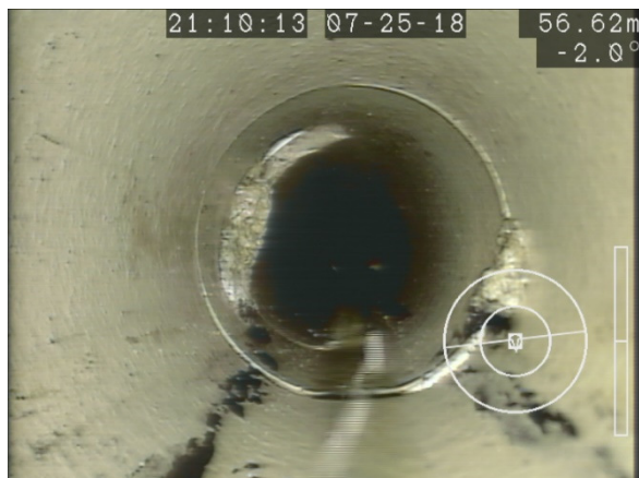
Figure 20: Calcite Buildup (56.6m from MH 34 towards MH 42)
