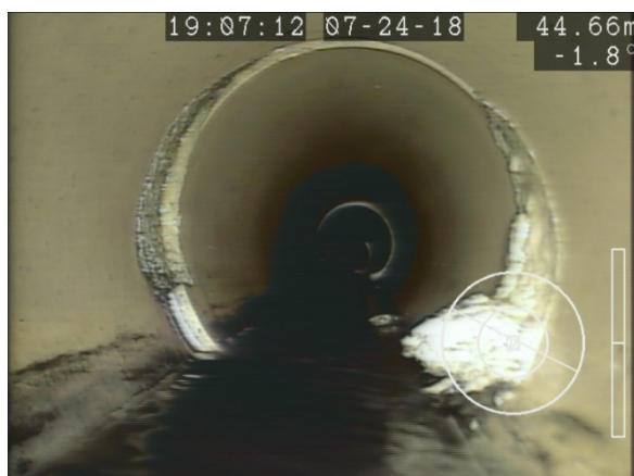
Figure 24: Calcite Buildup (44.66m from MH 28 towards MH 27)
