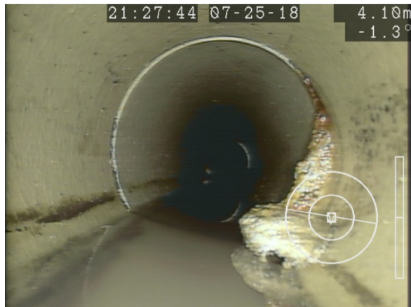
Figure 22: Calcite Buildup (4.1m from MH 42 towards MH 34)
