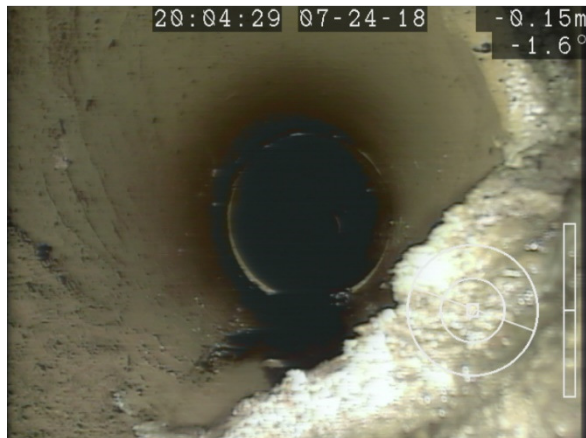
Figure 10: Calcite Buildup (at MH 24)
