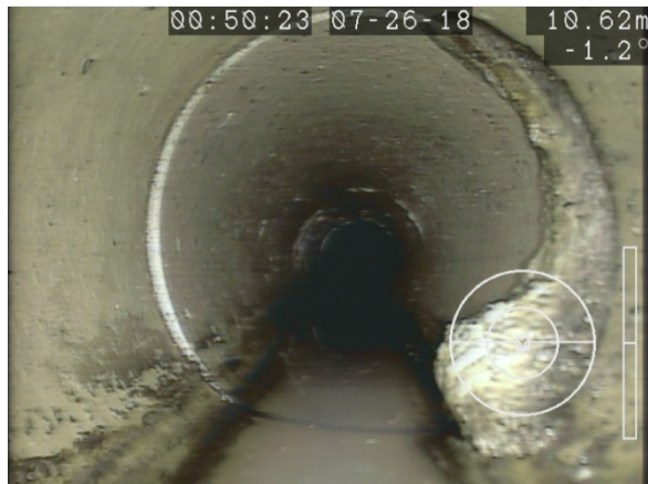
Figure 16: Calcite Buildup (10.6m from MH 31 towards MH 32)
