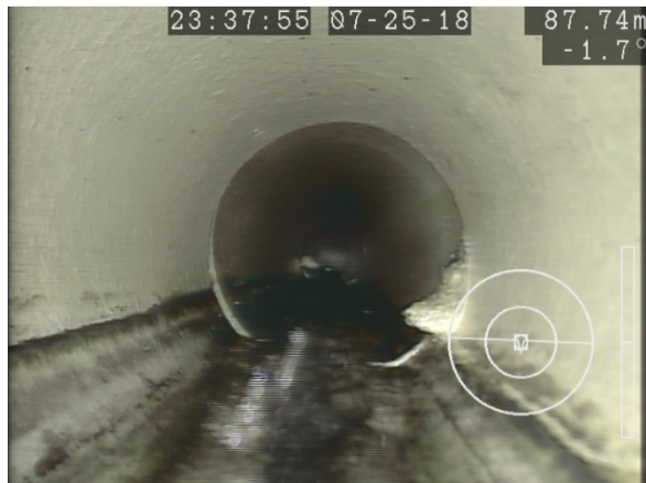
Figure 19: Calcite Buildup (87.74m from MH 33 to MH 32)
