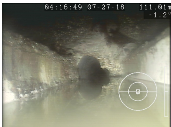
Figure 12: Calcium Buildup (MH 44)
