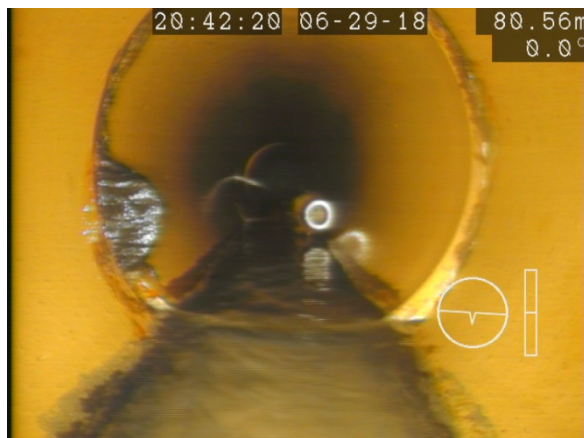
Figure 14: Calcite Buildup (81m from MH 4 towards MH 3)
