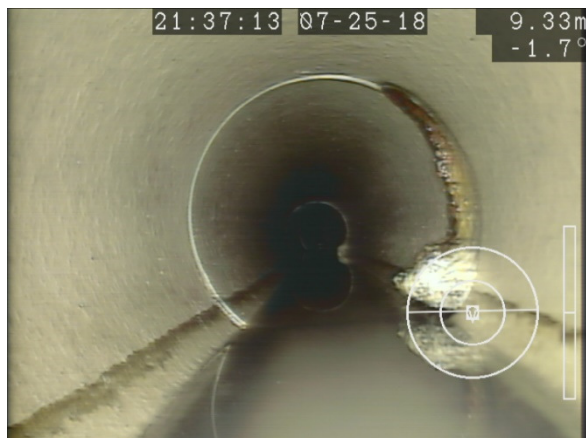
Figure 23: Calcite Buildup (9.33m from MH 42 towards MH 38)
