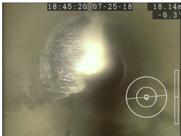
Figure 26: Calcite Buildup (18.14m from MH 39 towards MH 40)
