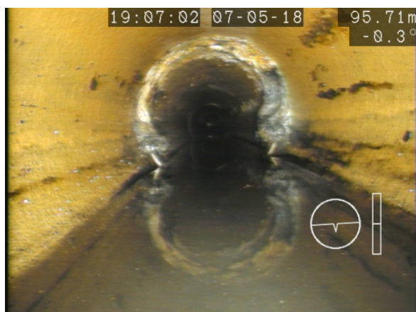
Figure 30: Calcite Buildup (95.71m from MH 18 to MH 29)
