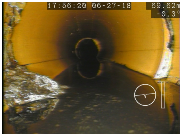
Figure 4: Calcite Buildup (69.62m from MH 16 towards MH 17)
