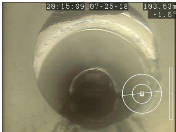
Figure 29: Offset in Pipe Just Outside Manhole (MH 35)
