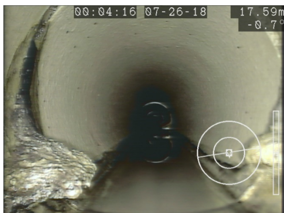
Figure 18: Calcite Buildup (18m from MH 32 towards MH 33)
