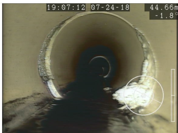
Figure 24: Calcite Buildup (44.66m from MH 28 towards MH 27)
