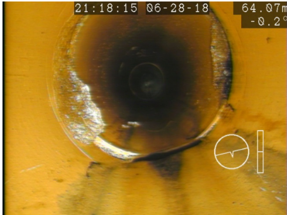
Figure 1: Calcite Buildup Blocking Camera (64m from MH 7 towards MH 6))
