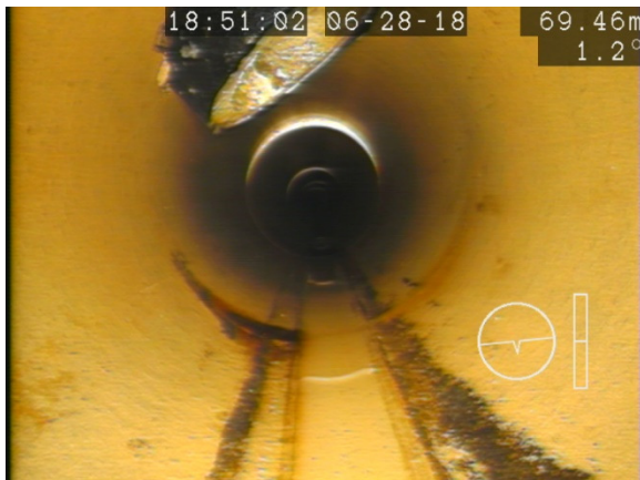
Figure 2: Extended Service (69.5m from MH 9 towards MH 10)
