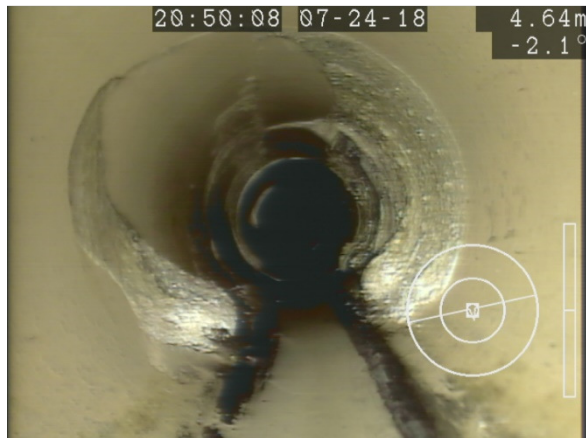
Figure 7: Calcite Buildup (4.6m from MH 23 towards MH 22)
