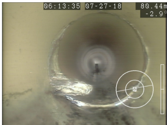
Figure 11: Calcite Buildup (80.5m from MH 43 towards MH 19)
