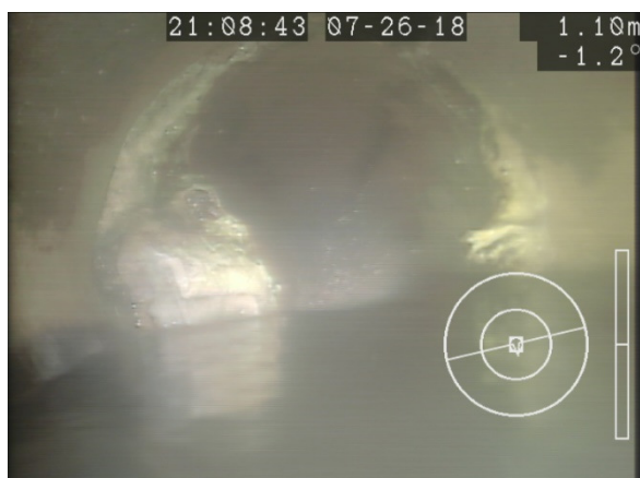
Figure 33: Calcite Buildup (at MH 26)
